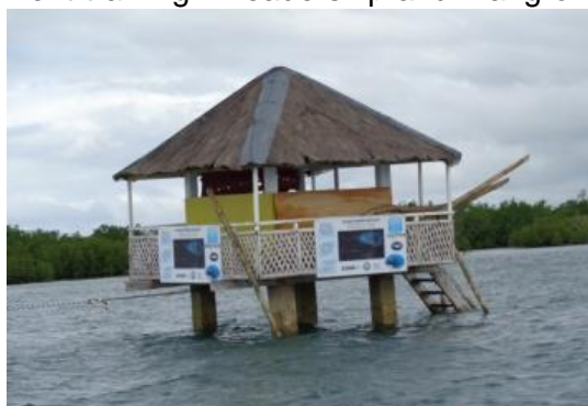
The repaired Matabao MPA guardhouse, Tubigon, Bohol.
